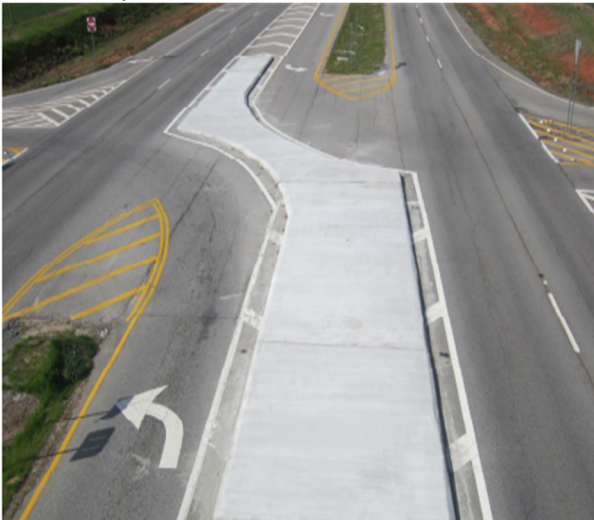
A Reduced Conflict U-Turn (RCUT) intersection example along State Route 20 in Henry County
